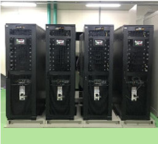
Hangang Mechatronics, a SolarEdge Critical Power partner in Korea, together with SolarEdge, came up with the answer – four SolarEdge 300KVA modular UPS systems in parallel, providing 1.2MW of real online power back-up with Li-ion batteries.
